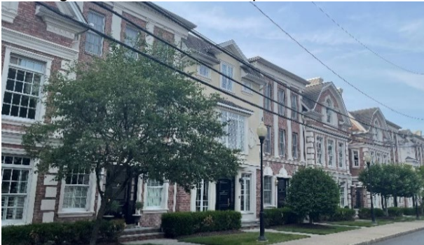
An example of potential viewshed from Bloomfield Avenue corridor
